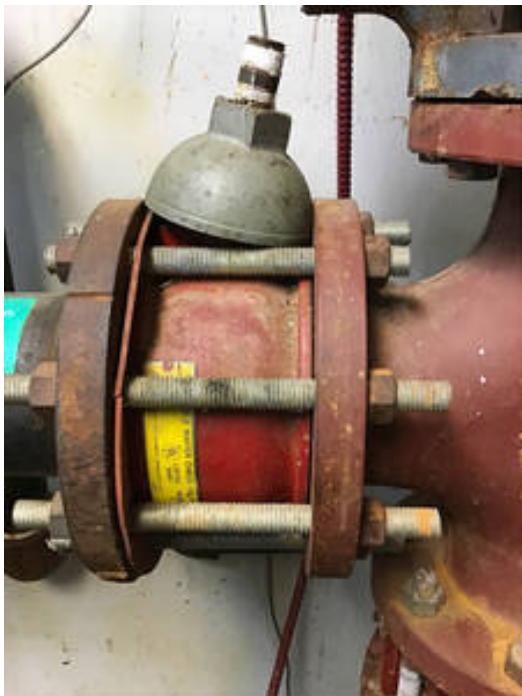
Valve - 4" Wafer Style Check Valve on FDC Sprinkler Room
