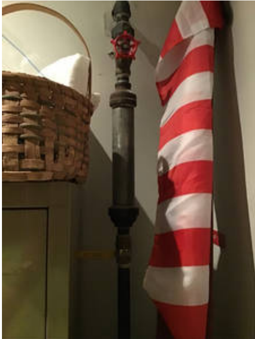
Drain Valve - 1/2" Low Point Drain Valve 2nd Floor - Air Compressor Room
