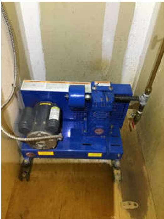
Drain Valve - 1/2" Low Point Drain Valve 2nd Floor - Air Compressor Room
