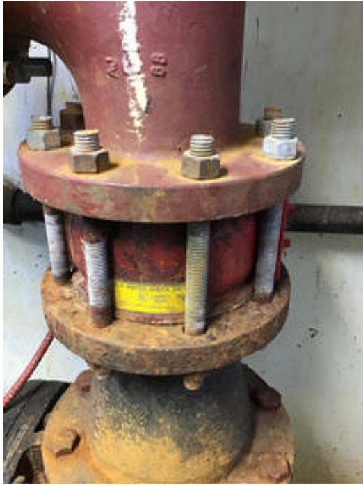
Valve - 4" Wafer Style Check Valve on FDC Sprinkler Room
